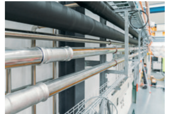
↑ Economical and corrosion-resistant system for cooling lines.
